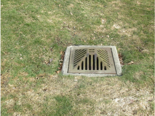
Erosion at catch basin (behind Unit 2700 shown)
