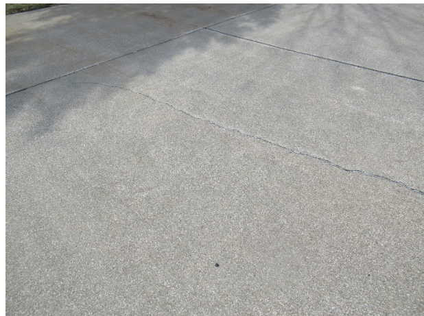
Access drive crack
