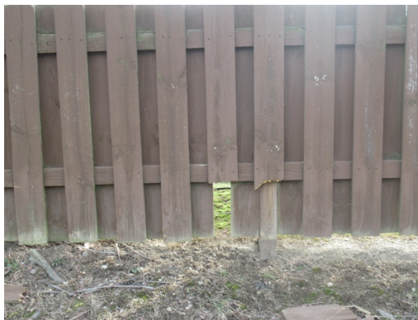
Damaged picket
