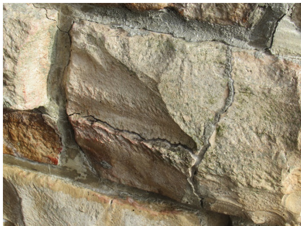
Masonry crack
