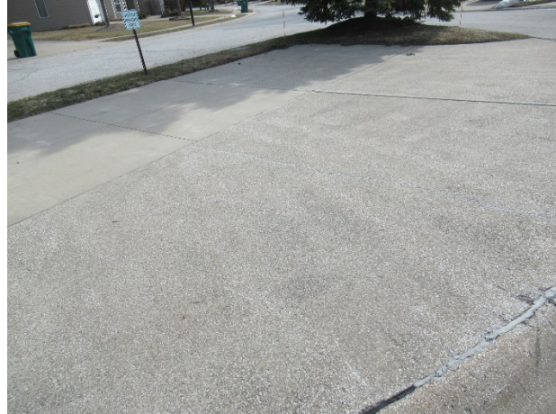
Parking area (note spall)
