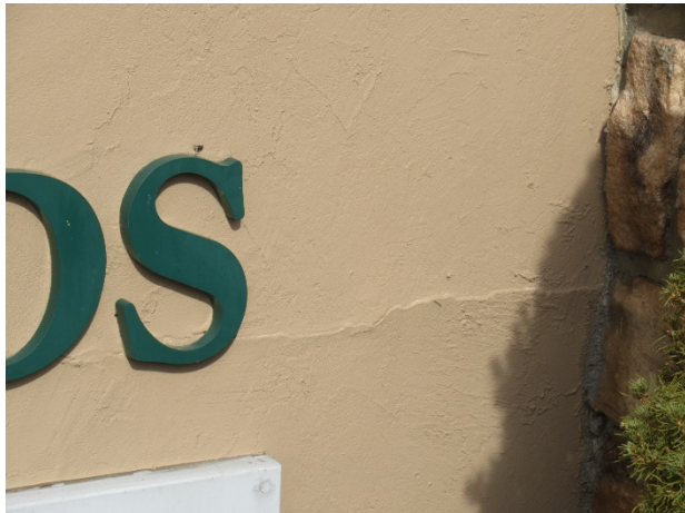
Signage crack (painted over)
