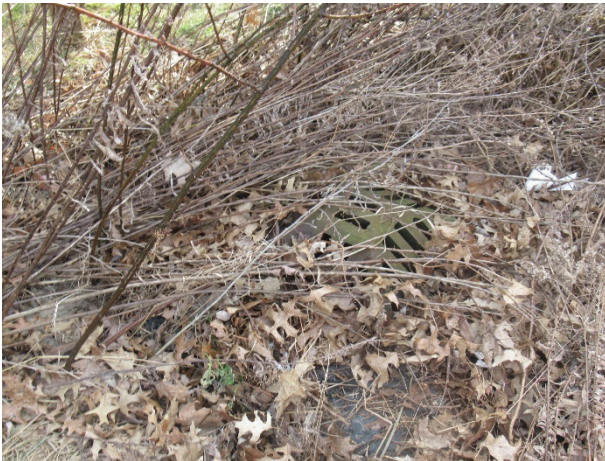
Erosion around catch basin (note partially covered by foliage)
