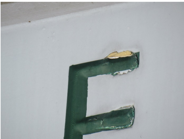
Finish deterioration at signage
